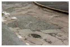
detection into a failing road surface as it is likely to fail again after a short time. For this reason it is common to have a policy that a SCOOT detector re-cut is not permitted if a road surface is failing, or if the area is due for resurfacing or remodelling within the next two years.
